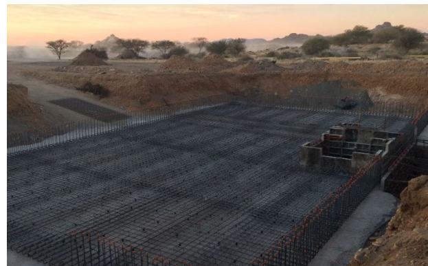
Phase 2 floatation plant under construction
